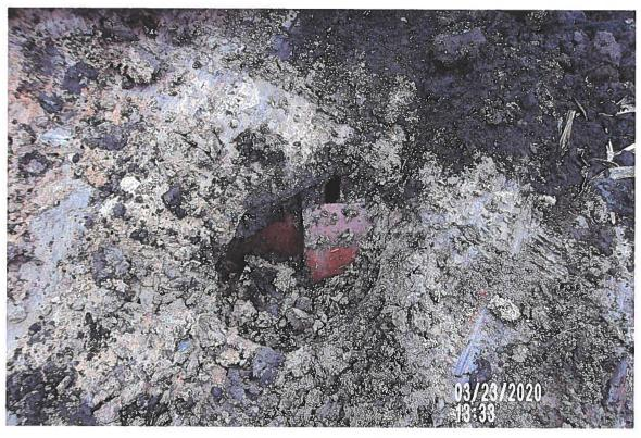
PILTURE# 3137 15 LOOKING SW SHOWING I" WIDE JOINT WITH JUST CLAY CHUCKS OVER JOINT ON MAIN JUST SOUTH OF 6" CONCRETE TILE TIEIN.
